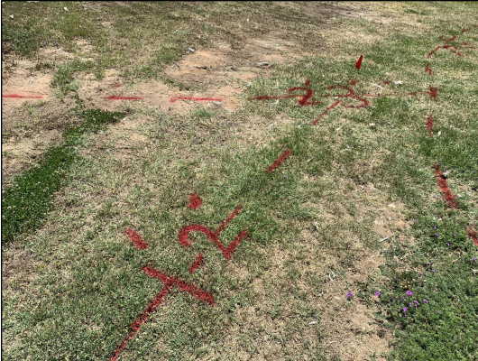
Several electrical lines intersecting
